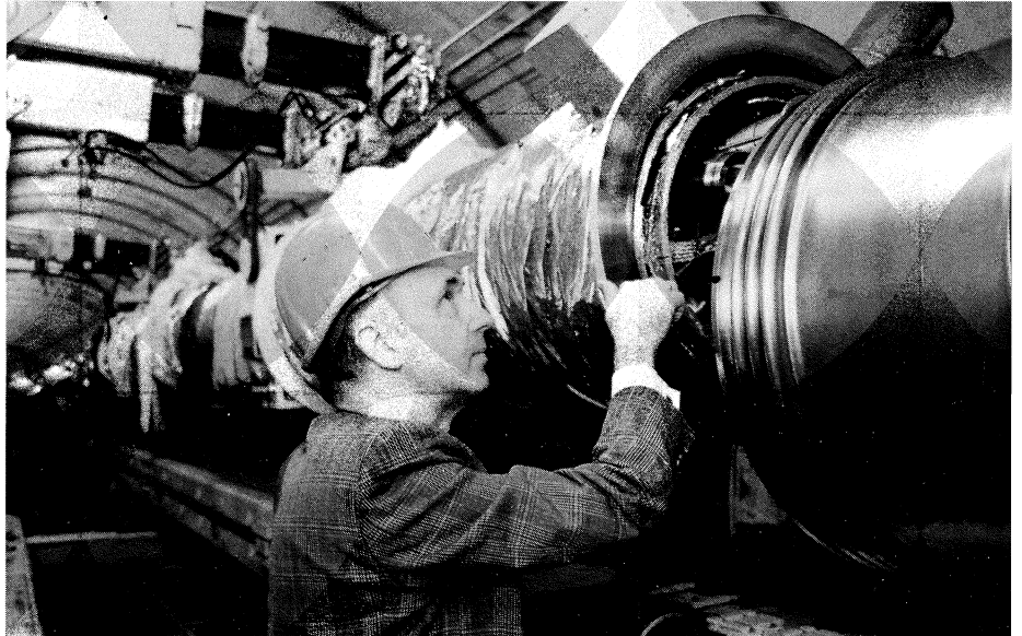
▲ 19 September – DESY Director Volker Soergel watches as the last of the 646 superconducting magnets moves into position in the proton ring of the 6.4 kilometre HERA electron-proton collider.
